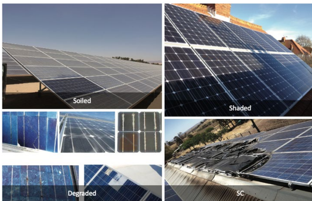
Figure 1: Photos of PV arrays containing the four most common faults [1].
