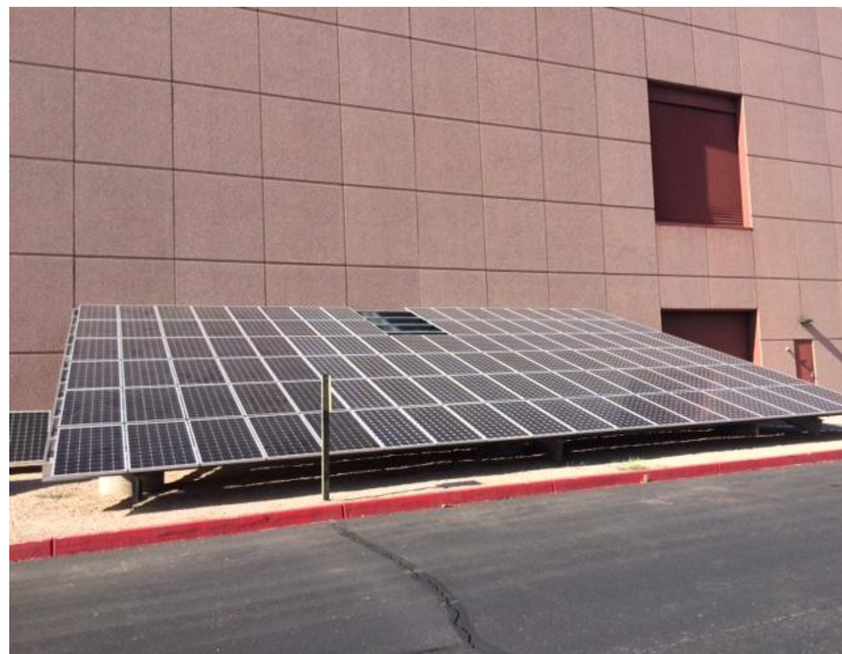
The SenSIP 18kw (104 panel) experimental facility established at ASU with industry collaborators [3].
