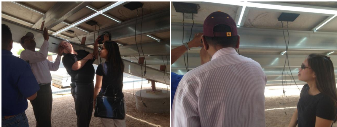
Fig. 4. Personnel from our GOALI partner ViaSOL inspecting the facility in June 2015.
