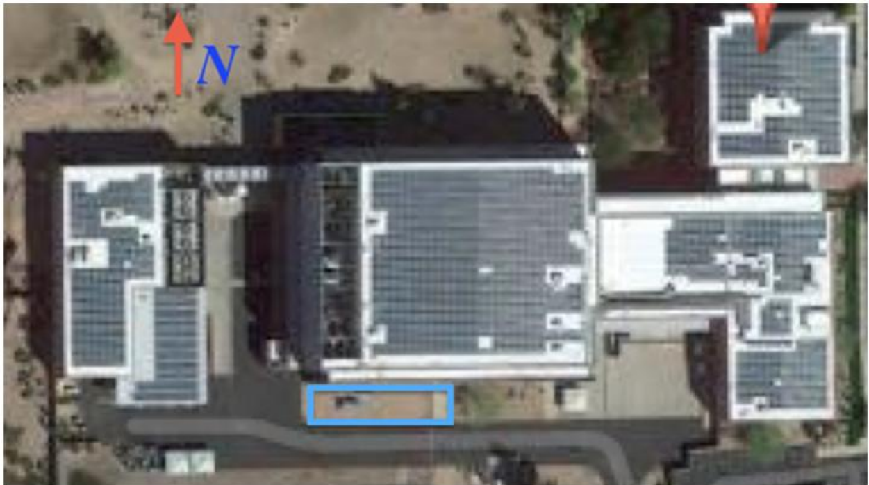
Fig. 1. ASU Research Park in Tempe. aka Micro Technology Works (MTW). Area in blue is where the Solar panels were installed. 104 panels were installed as shown in Fig. 2.
